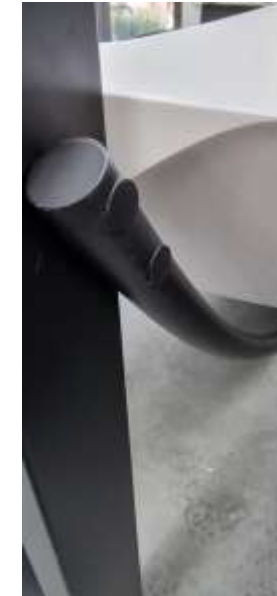
Curved brace connected to steel frame
